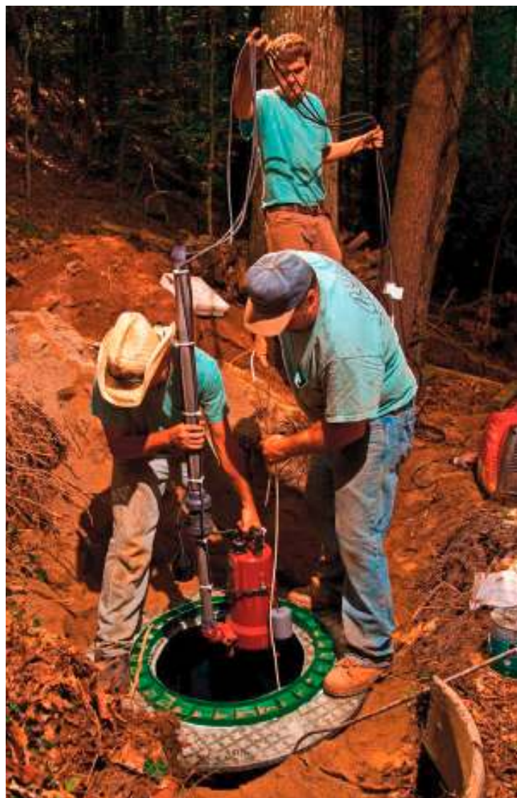
With Justin Kilgore keeping electrical lines under control, Heath (left) and Harold Kilgore lower a Liberty Pump into a grinding station in Blue Ridge, Ga.
